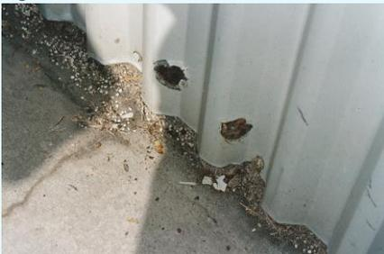
accelerate the corrosion of COLORBOND® prepainted steel, COLORBOND® Ultra prepainted steel and ZINCALUME® aluminium/zinc/magnesium alloy-coated steel.
