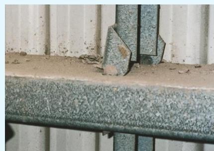
Furthermore, the purlins should be post-painted with an appropriate high-build industrial paint system as recommended by a reputable paint supplier.
